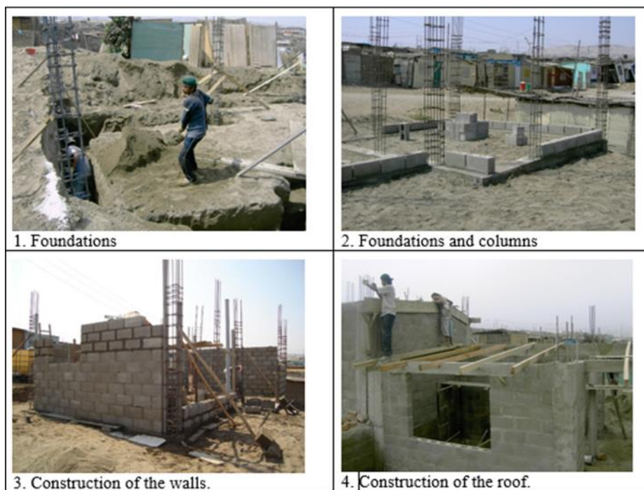
Figure 11 Concrete structures for houses to be earthquake resistant
